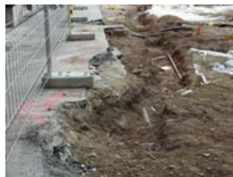
PIC02508 rasa serveis a Sector 2
