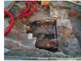
DSCN2111 Esc 3 Vista general
