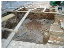
DSCN1325 Vista general bunker
