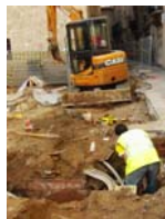
PIC02507 Rasa serveis a Sector 2
