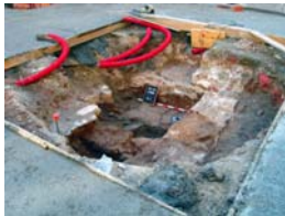
DSCN2114 Esc 3 Vista general
