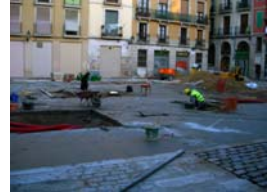
DSCN2101 Vista general
