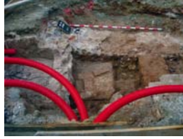
DSCN2097 Esc 3 Vista general
