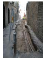
DSCN1369 Vista general
